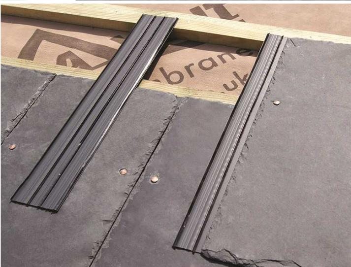
Eliminates the angle of creep and allows slates to be laid on a roof with a pitch as low as 12 degrees.
