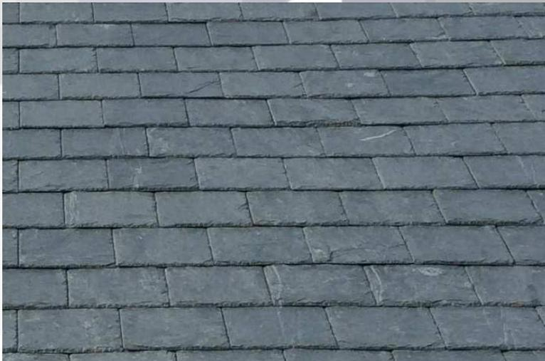
Samaca Q53 is a dark blue grey slate produced in the Los Molinos region of Northern Spain. The slate has a good natural texture giving the appearance of a domestically quarried slate to the finished roof. The duller texture of the slate is in contrast to many imported slates which can have a very noticeable sheen on the roof.
